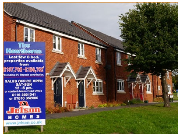
Figure 10: Flint Drive, Asfordby
