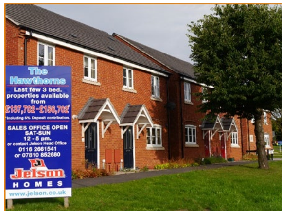
Figure 10: Flint Drive, Asfordby
