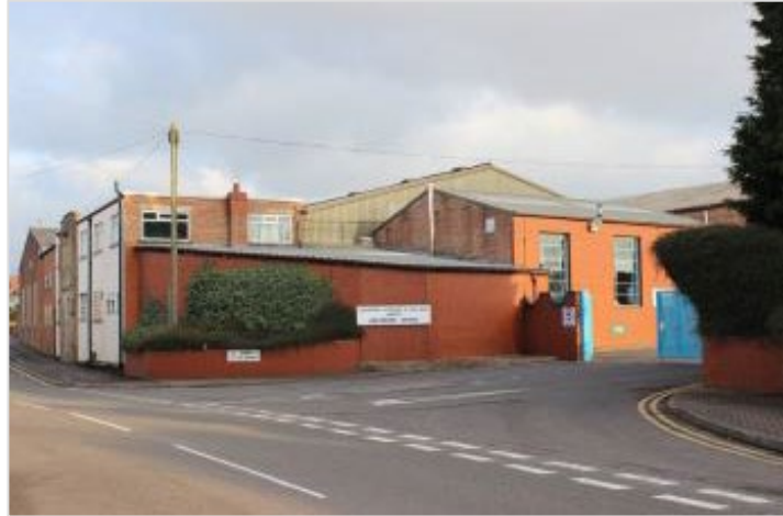
Figure 12: Asfordby Storage and Haulage Depot, Main Street, Asfordby
